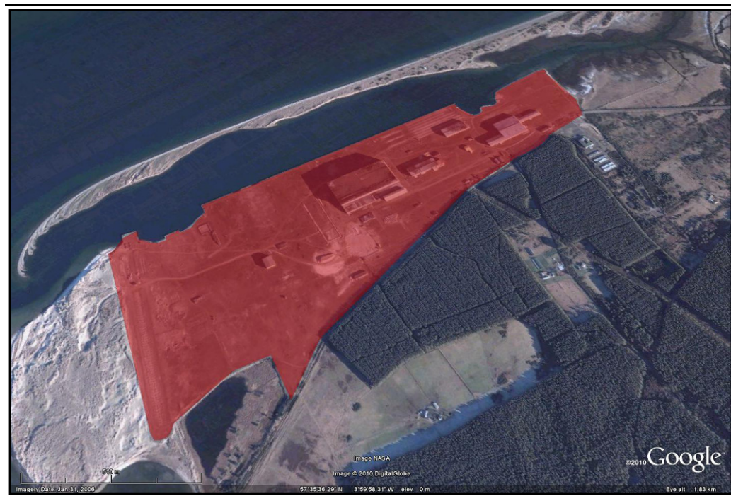
Figure 6.4 Aerial View of Ardersier
